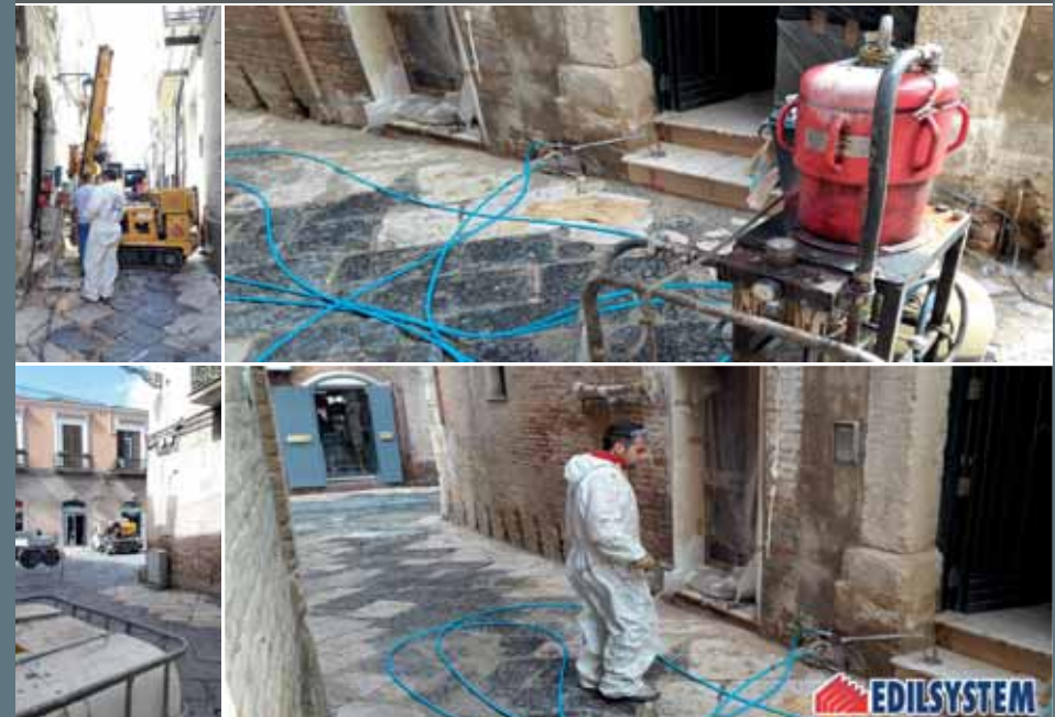
Condominio C.So Garibaldi- Lucera (FG)
